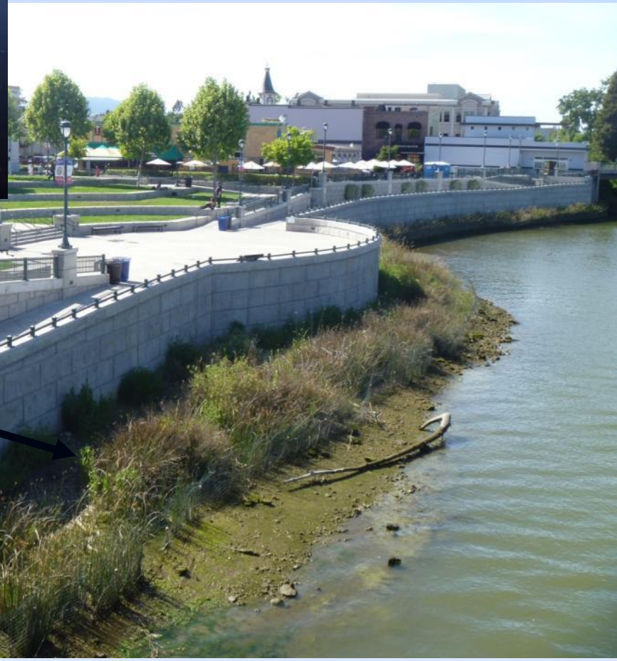
Veterans Park Floodwall 2014
