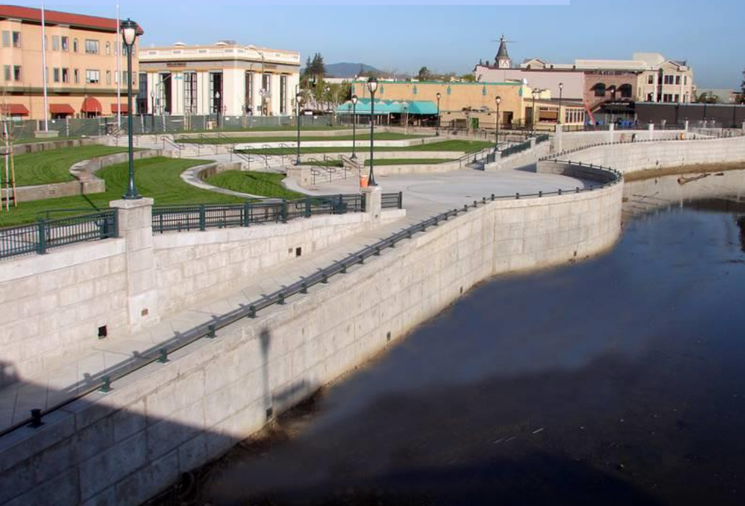
Veterans Park Floodwall 2008
